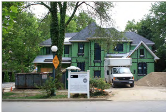
New infill construction in progress on Victoria Lane
