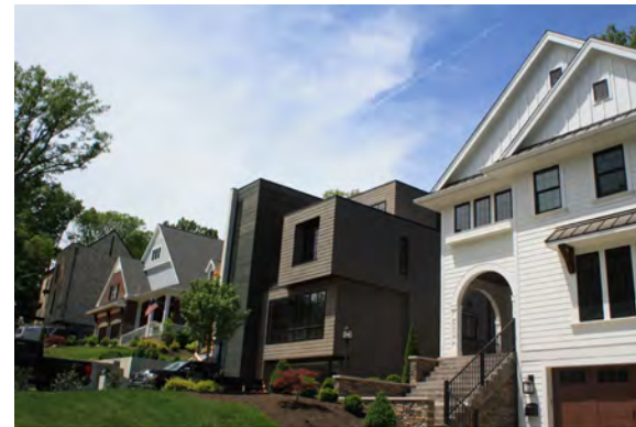
Four new single-family homes on Menlo Avenue
